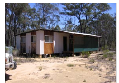
Phelps Hut in Durridgere State Conservation Area
